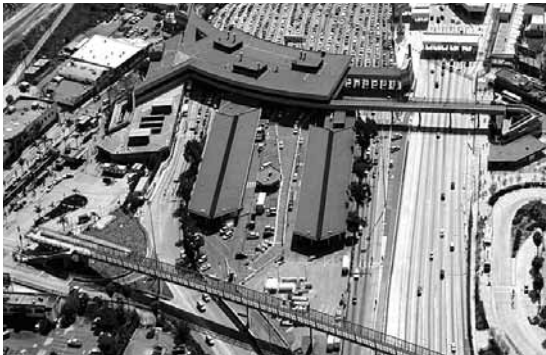
An example of AMG Demolition's ability to complete challenging jobs includes this $7 million project at the world's busiest border crossing in San Ysidro, Calif.
