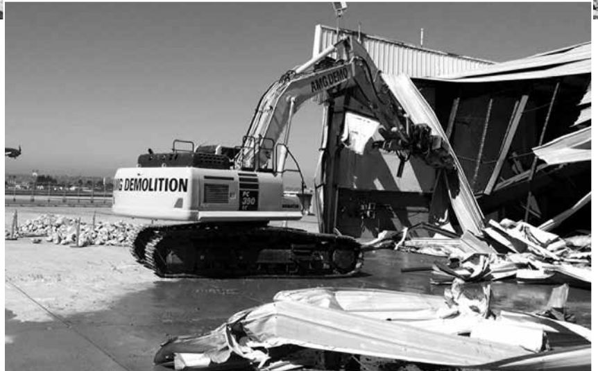
An AMG operator uses a Komatsu PC390 to tear down a hangar at Landmark Aviation at the San Diego Airport. "Since we got the PC390s earlier this year, they've become our workhorse excavators," said Estimator Mike Gafa Jr. "Our operators love them."
