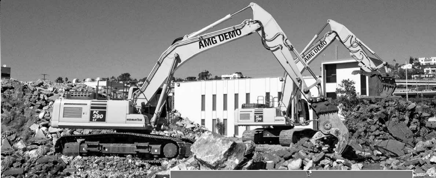
AMG Demolition recently purchased these two Komatsu PC390LC-10 (90,000-pound) hydraulic excavators.
