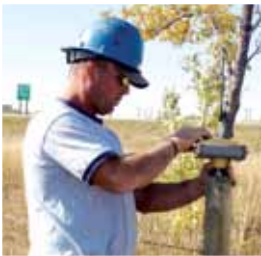
Brad Schoenfelder sets up a Topcon 3D-MC 2 base unit used to set grade via GPS with a Komatsu D51 dozer. Schoenfelder Construction shaved months off a site-work project with the Topcon/Komatsu combination.
