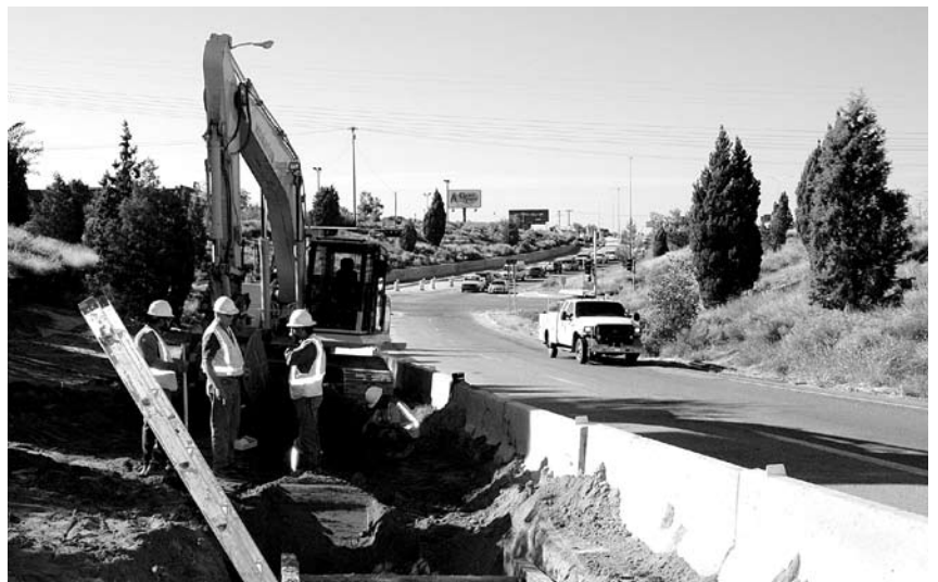
Underground contractors know good practices in trench safety are extremely important, including trench shields or boxes for deep excavations, ladders for egress at proper intervals and hard hats and other safety gear to keep workers protected from potential falling objects.
